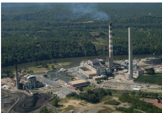
Coal-fired electrical generating plant
