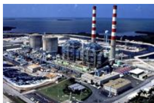
Electrical Generating Plant
