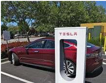
Tesla Supercharger Picture: Courtesy of Tesla
