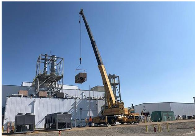
*Figure – Installation of New Chillers*
