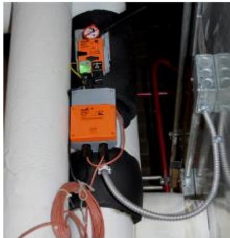
*The Belimo Energy Valve is an IoT cloud-connected pressure independent valve that monitors coil performance and energy consumption while maintaining Delta T.*
